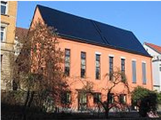
Solar panels on rooftop
