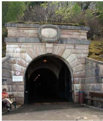
Directing structure (tunnel)
