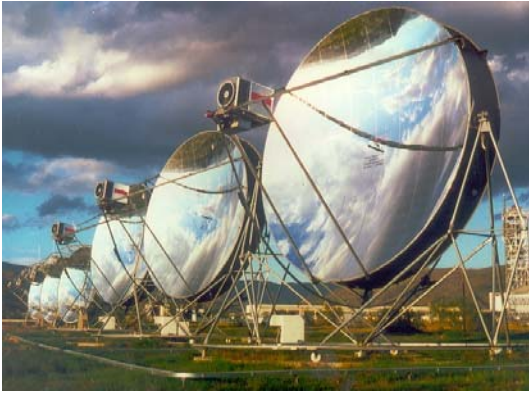
Parabolic dish used to produce solar power
