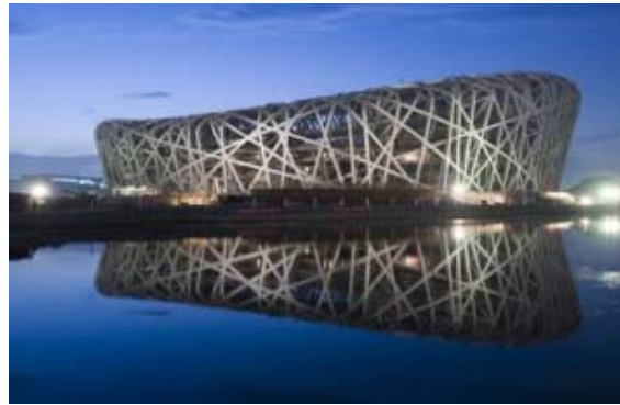
Sheltering structures (Bird Nest or Beijing National Stadium. Principle design firm: Herzog & de Meuron of Switzerland)
