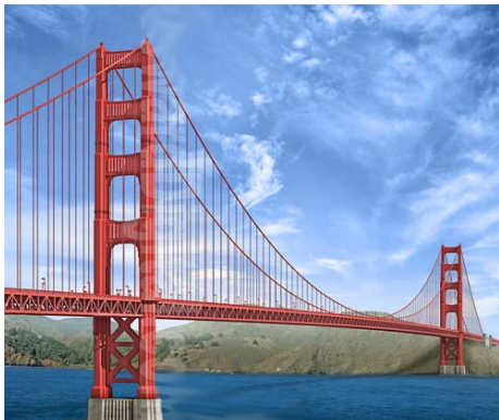
Transportation structures (suspension bridge)
