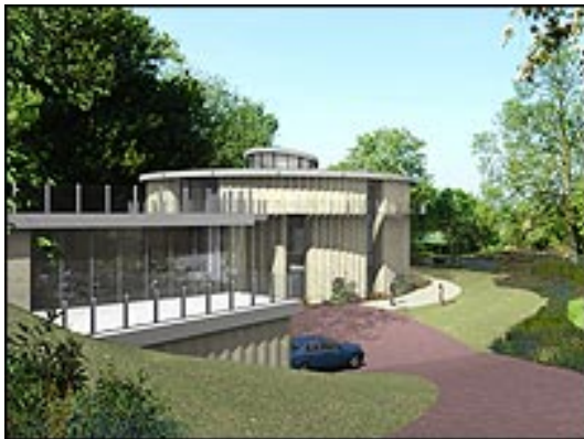
Figure 11. Solar-powered building that can rotate on wheels and tracks, invented by Hamilton, a British inventor (BBC Chinese, April 13, 2007. Retrieved January 30, 2009, from http://news.bbc.co.uk/hinese/trad/hi/newsid_6550000/newsid_6554500/6554549.stm )
