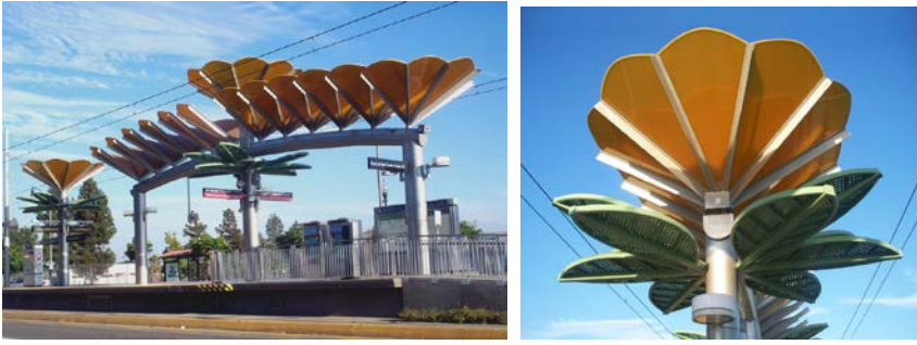
Figure 3S. Flower petals and leaves make the roof of the Gold Line Atlantic Station.
