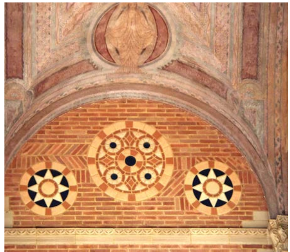
Figure 1J. Wall decoration with brick pieces of different colors in a research building at UCLA.
